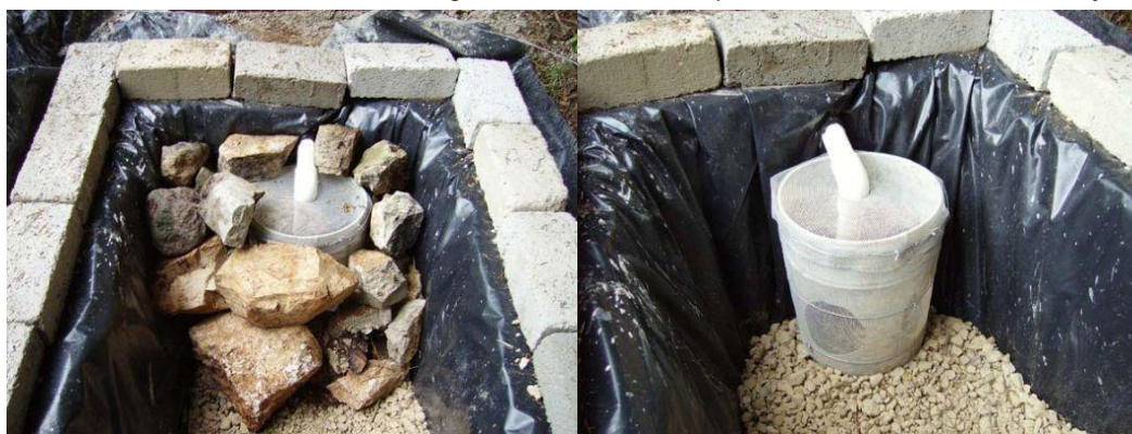
Fig (2) multi-layer filter of the household treatment system.
