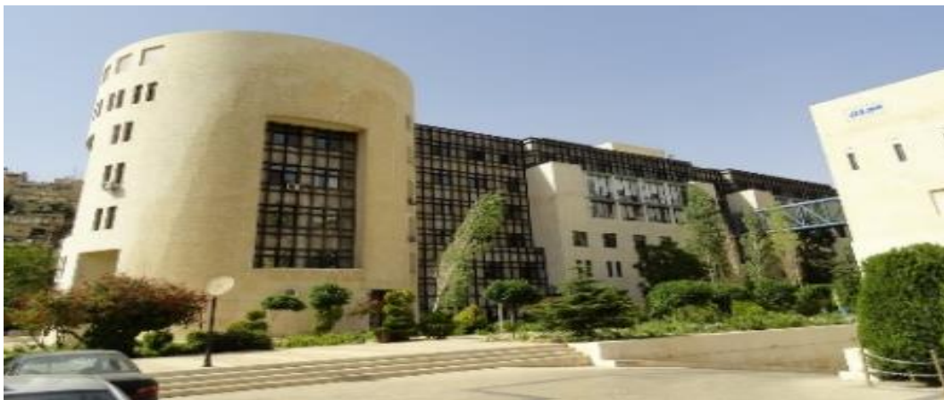
Figure (12) City Hall of the Greater Amman Municipality (Google)
